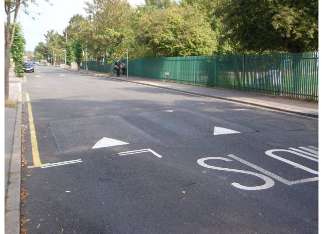
Photograph MW9: Sydenham Road, view north
